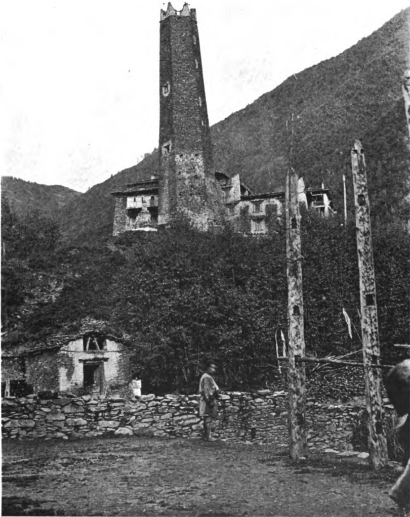
A MANTZE CASTLE AND TOWER; KIAKOS (ON RIGHT) FOR DRYING CORN.
